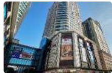
Ba Trieu Office Building
